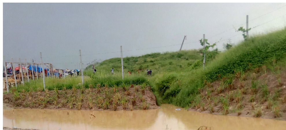
Another ecosystem service is provided by short grasses and shrubs on a slope, preventing soil erosion because the vegetation helps to hold on the soil in the steep slope.
