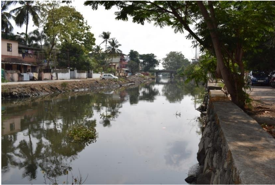
Figure 16: Thevara Canal which has been encroached upon
