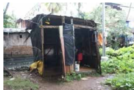
Figure 7: Slum toilets along the St. Inez Creek
